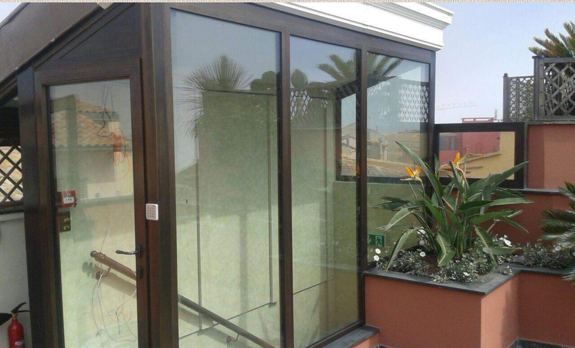
Veranda in Architectural Bronze. Door with automatic opening and smoke detector.
